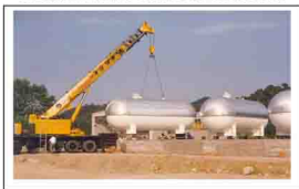
50 m 3 . NH3 LIQUIFIED SERVICE PRESSURE 22 bar
